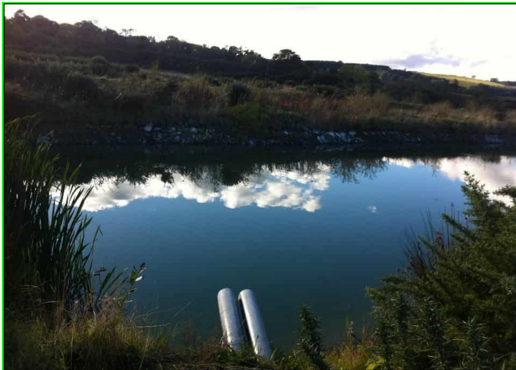
Plate 7-1 Existing Lagoon at Ballinclare
