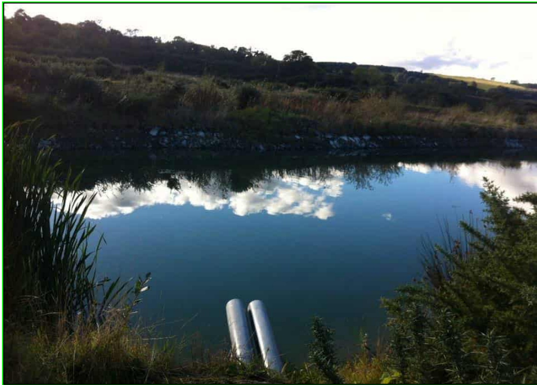
Plate 7-1 Existing Lagoon at Ballinclare
